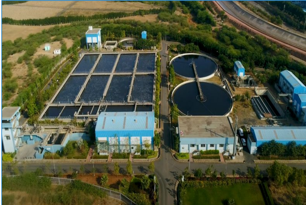
Welspun STP – 40 MLD located in Anjar , Kutch
